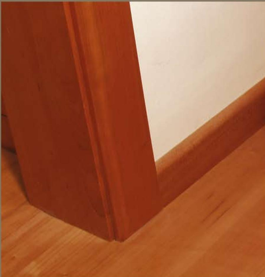
The Perfilstar door frame allows you to hide the uncut head of the skirting because the width of the skirting became hidden in the door frame.
